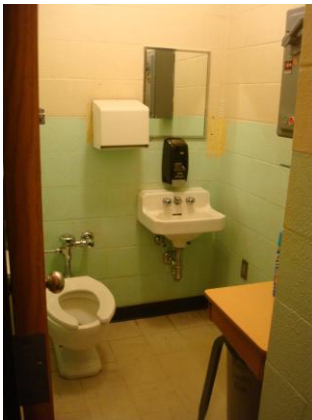
NON ACCESSIBLE TOILET ROOM
