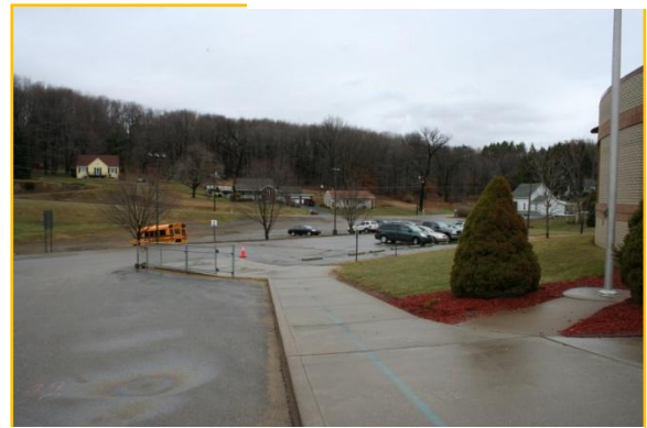
LACK OF HANDICAPPED ACCESSIBLE PARKING
