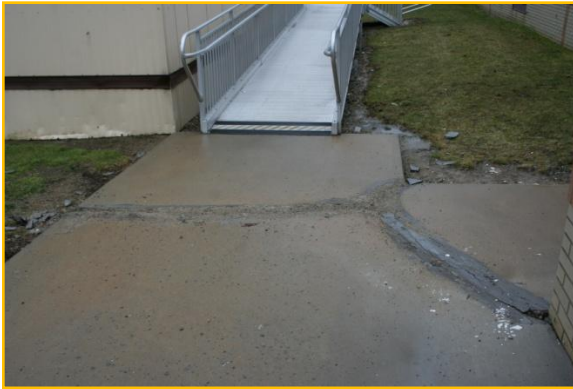
EXTERIOR CONCRETE AT MODULAR CLASSROOM
